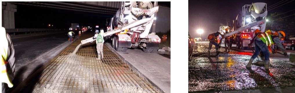
Figure 1- BCSA concrete placement on Mexico City- Queretaru highway.
