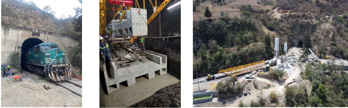
Figure 3- BCSA concrete placed on the Puebla-Veracruz railway tunnel, Mexico
