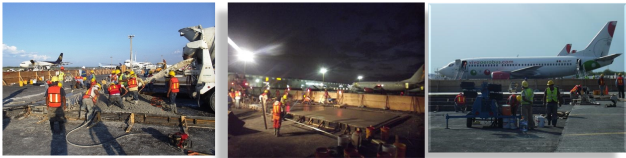
Figure 2- BCSA Concrete placement at the Monterrey International Airport, Mexico.
