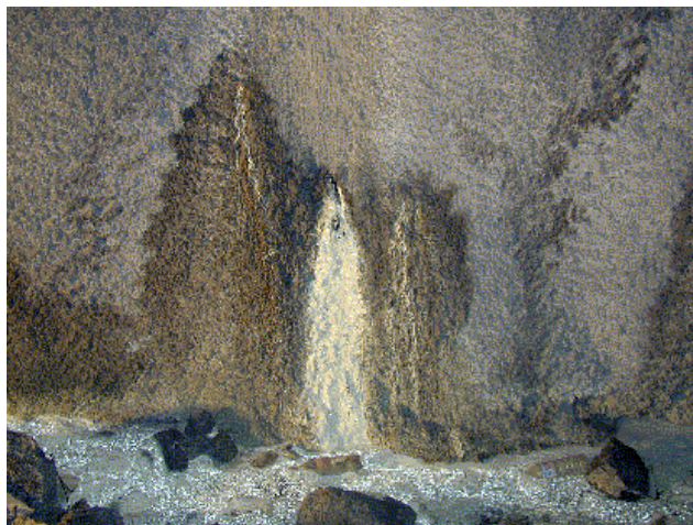
Figure 3. "Gotschna" tunnel: ground water locally penetrating the shotcrete lining. Depending on the amount of running water large amounts of biomass may form. The white mass in the center of the picture represents a colony of sulfur bacteria.
