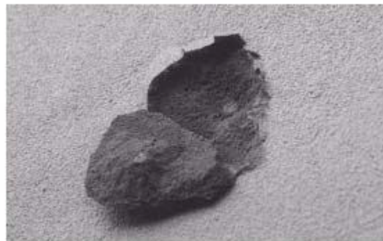
Figure 2. Pop, 40-mm in diameter, with nodule of about 5-mm diameter in centre
