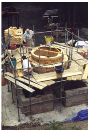
Figure 4. Construction in progress, central circular kiln shaft rising from concrete base built around circular wooden former and with early stages of square outer concrete block skin.
