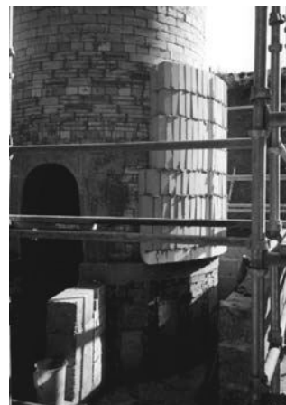
Figure 5. Completed double thickness brick kiln lining with beginnings of double thickness block insulation, resting on refractory concrete ring.
