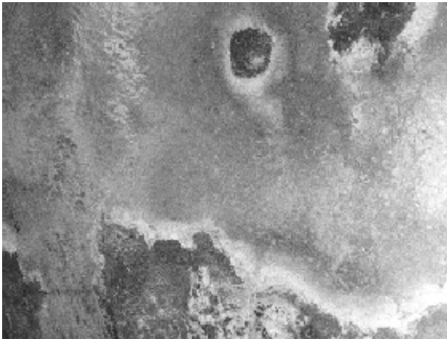
Figure 1. Shotcrete lining in the service tunnel "St. Gotthard" (upper part of the wall) showing a more or less uniform cover with bright efflorescence. Dark (wet) regions within the shotcrete mark localities with water transport and evaporation through the shotcrete.
