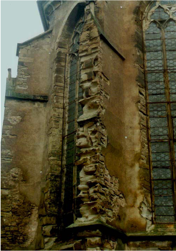
Figure 5. Zeitz cathedral damaged stone
