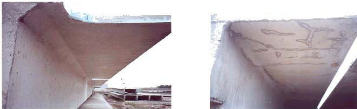
Figure 2. Comparison of two pre-stressed double “Tees” prepared by the same manufacturer with the same concrete formulation and cured under identical condition for the same period of time. The Tee on the left was prepared with the admixture and the Tee on the right was prepared without the admixture.
