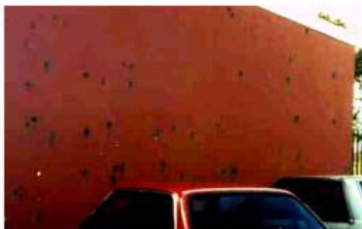
Figure 1. Typical incidence of pops in plaster
