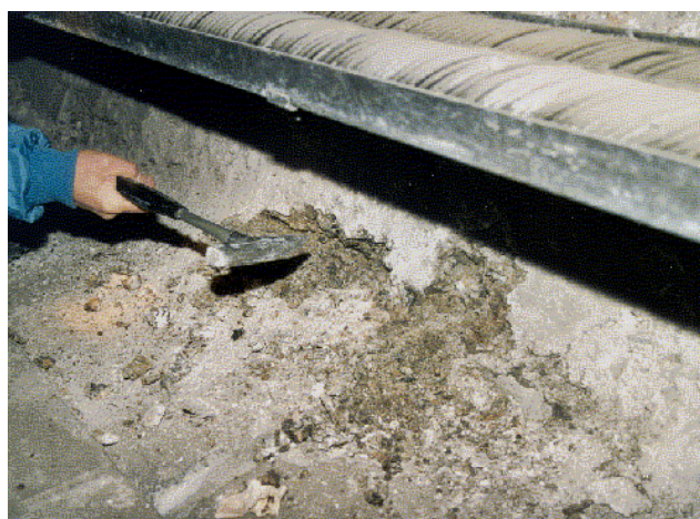
Figure 8. Concrete lining of “San Bernardino” tunnel: depending on whether the altered concrete is wet or dry it shows properties of a mush or a crumbly material.
