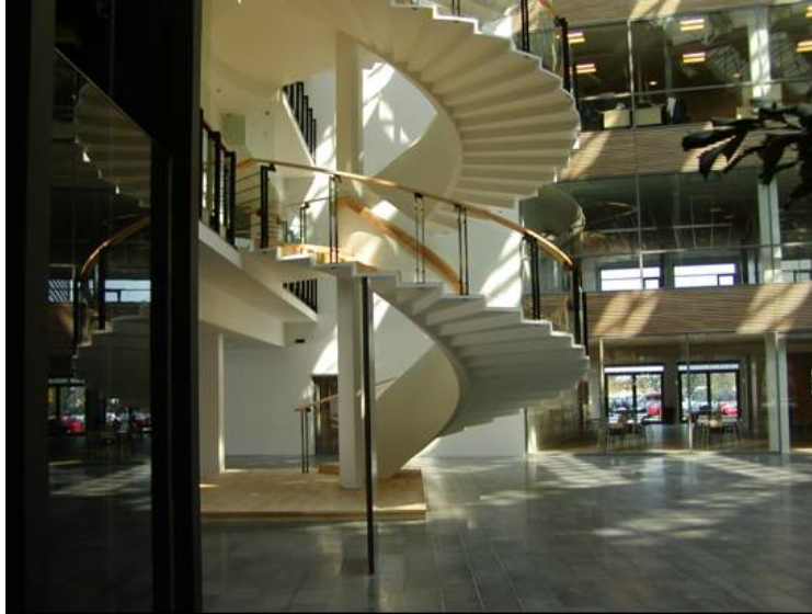
Figure 3: Spiral staircase with cantilevered steps produced in CRC.
