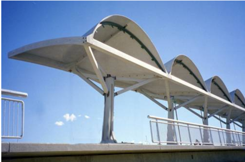
Figure 5: LRT Train Station (Calgary, Canada): 24 thin-shelled Ductal®-FO canopies
