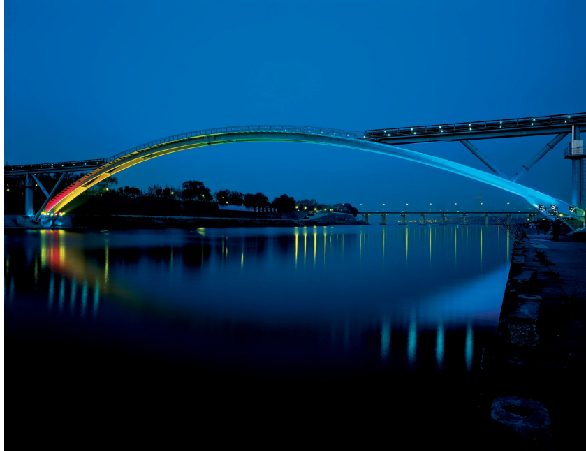
Figure 4: Seonyu Footbridge in Ductal® (2003, Seoul, Korea), architect : Rudy Ricciotti; photo: © Philippe Ruault
