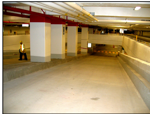
Figure 1b: Ramp after reconstruction
