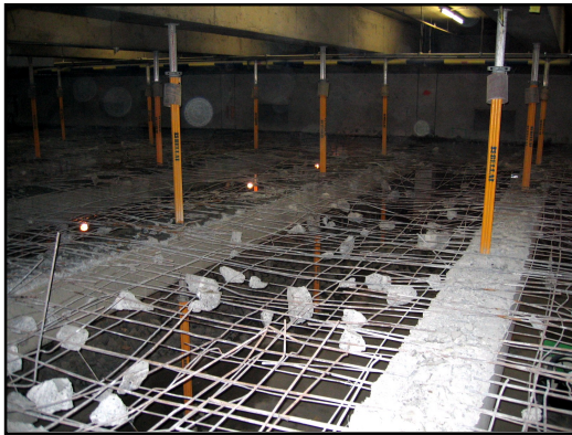
Figure 1a: Slab during demolition (before removal of reinforcement)
