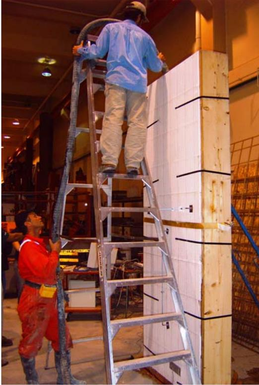
Figure 4 : Full-Height ICF Wall Cast
