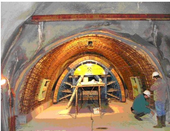
Figure 1: View into the tunnel construction area.
