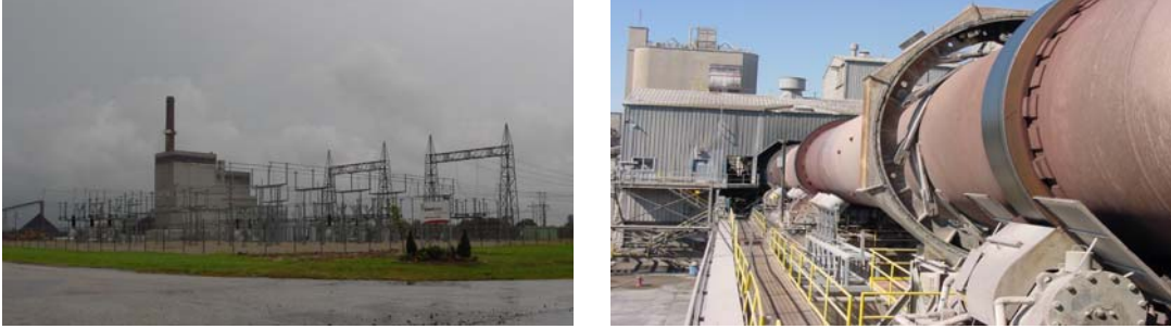
Figure 1. Coal-Fired Power Station and Cement Plant in the Midwest
