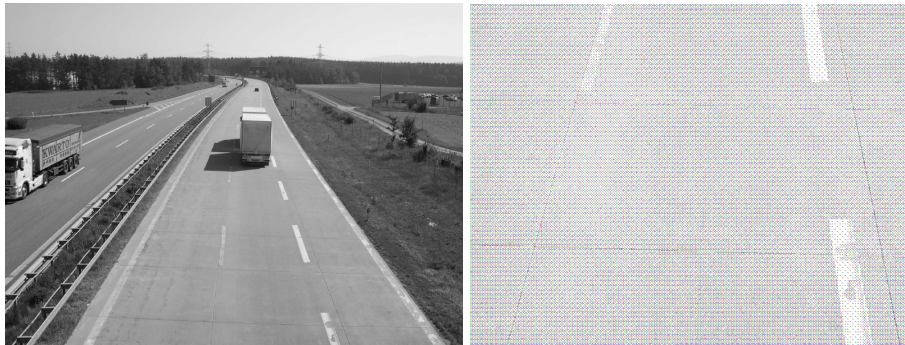
Fig. 1a: 9 years old concrete road produced with CEM II/A-LL in a region that is suffered by strong frost during winter time. The surface of the road is still in a very good condition. It shows neither cracks nor scaling or spalling.
