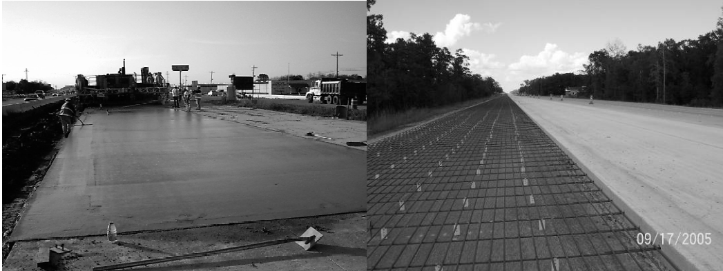
Fig. 3 Fresh (left) and hardened (right) concrete surface for Highway 69.
